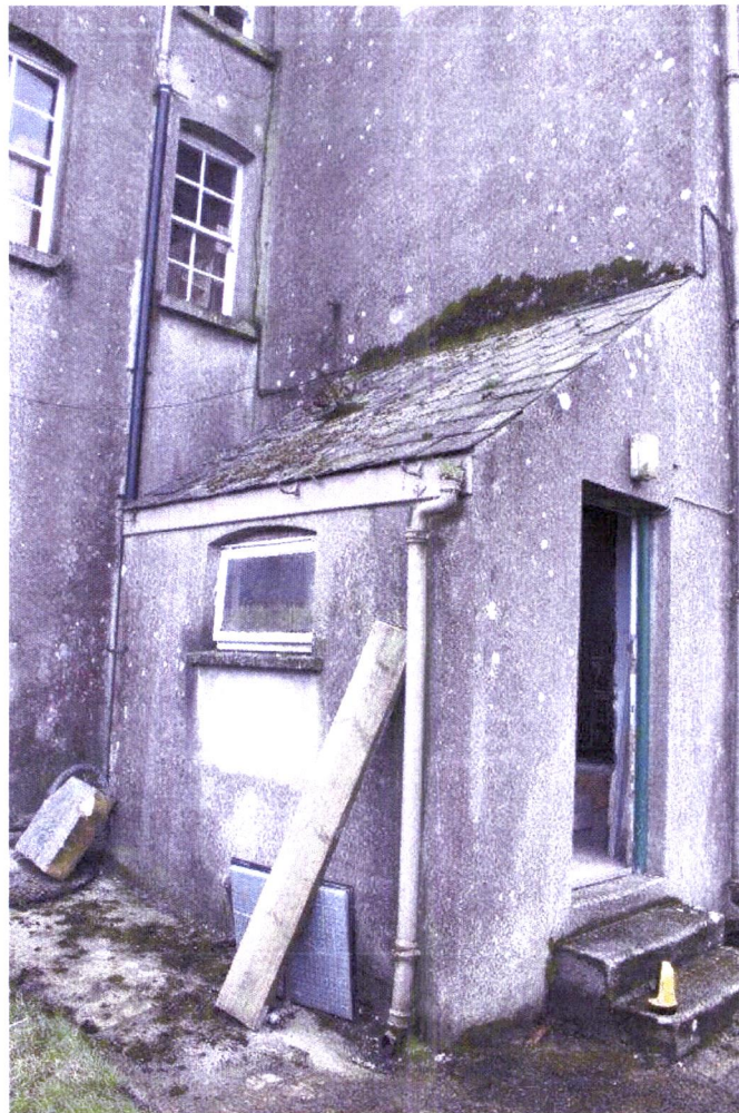
Figure 7: The rear extension. (9592)
