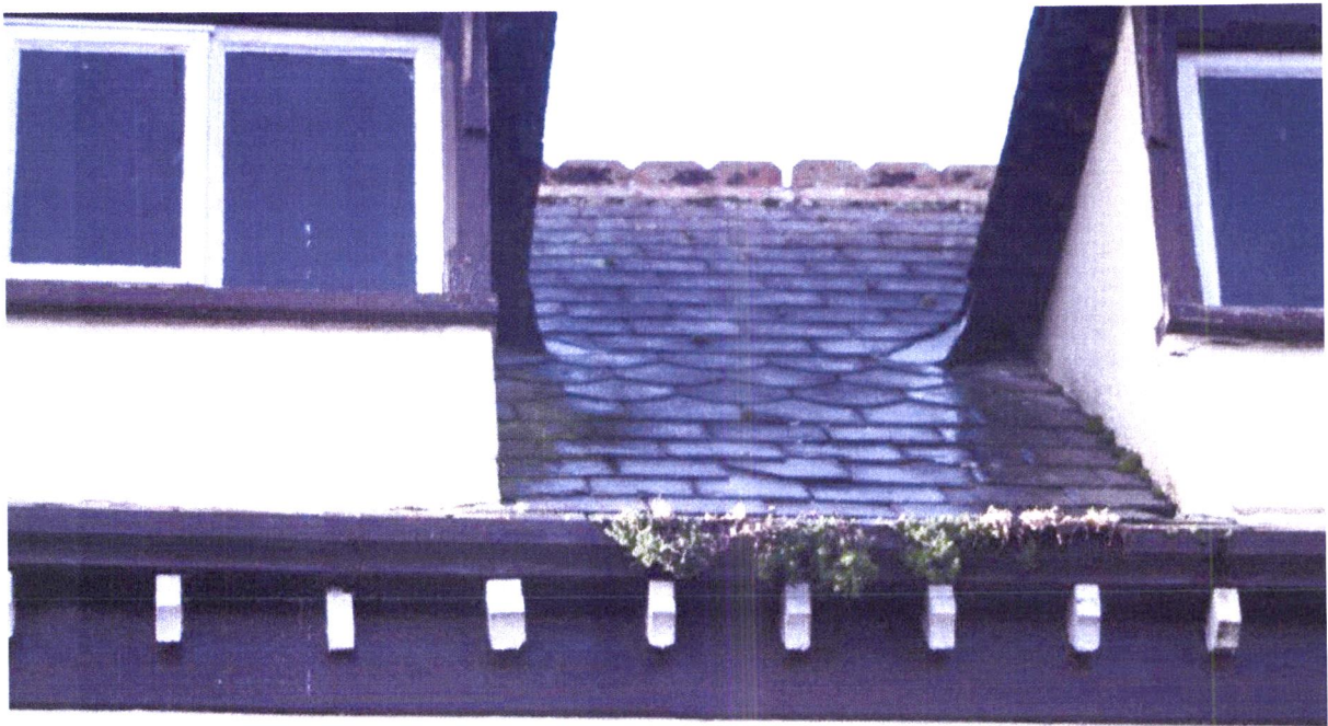
Figure 2: The southwestern end of the roof showing slipped, broken, re-fixed Blue Bangor slates and broken cast iron gutter also notice the three courses of round ended slates. (9654)
