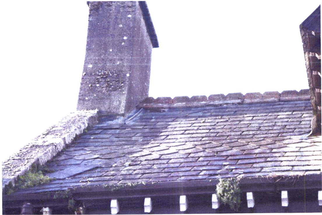
Figure 2: The southwestern end of the roof showing slipped, broken, re-fixed Blue Bangor slates and broken cast iron gutter also notice the three courses of round ended slates. (9654)
